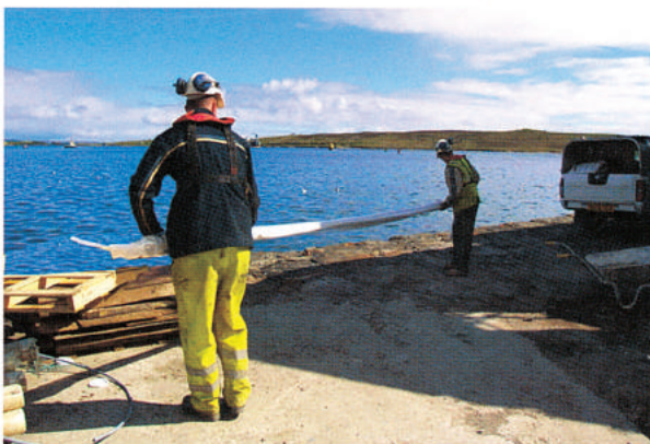
Cintec anchor being carried to the end of the quay ready for installation.
