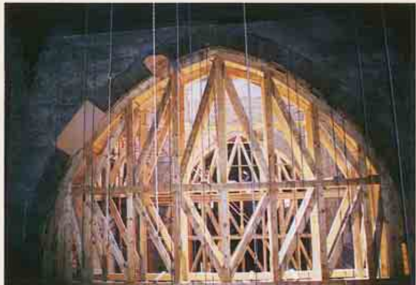
Temporary support of the Dikka arches
