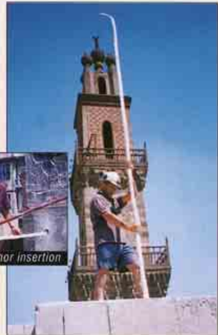
5 metre long vertical anchors at roof level
