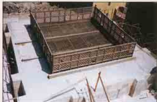
Roof section above central courtyard
