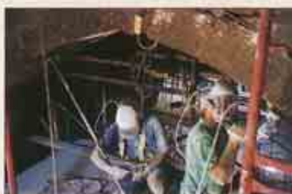
Diamond drilling the arch stones
