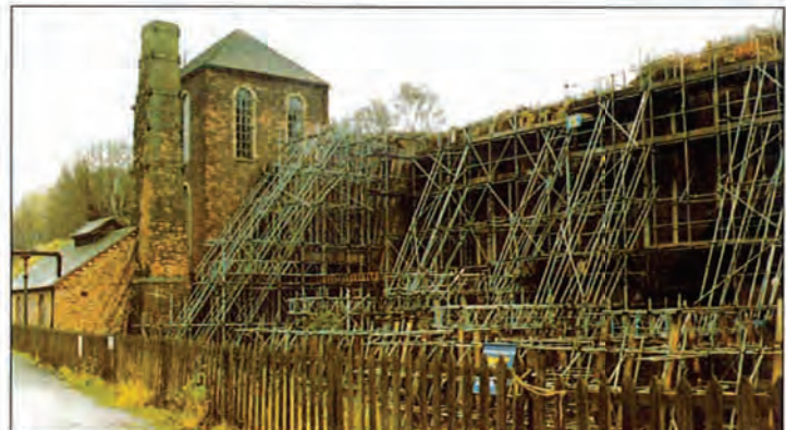
Restoration work in progress
