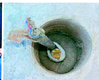
Injected vertical anchor
