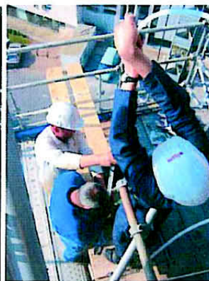
The installation of a vertical anchor
