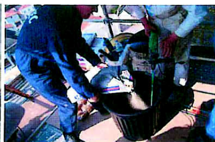
Preparation of grout
