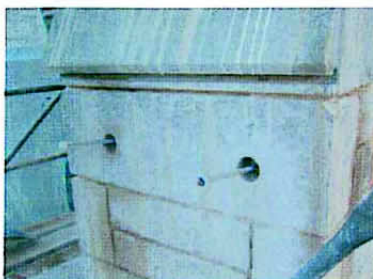
Horizontal anchors ready for injection
