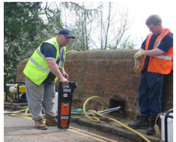
Checking for sub-surface services during bridge survey.
