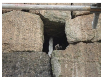
Pre-injection with masking tape
