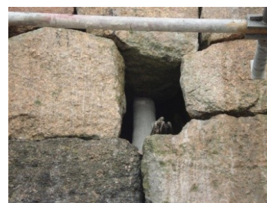
Anchor grouted & expanded
