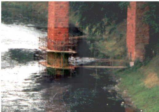
View of drilling platform
