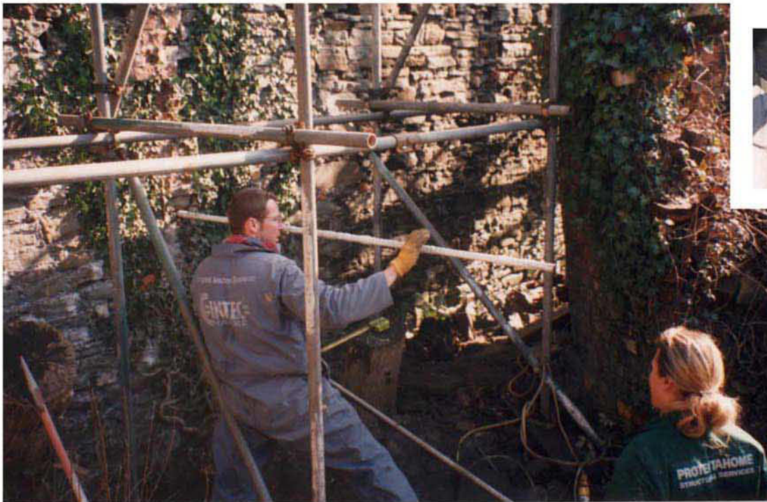
Insertion of 3m Cintec Anchor (left), and its inflation using cementitious grout, (above).
