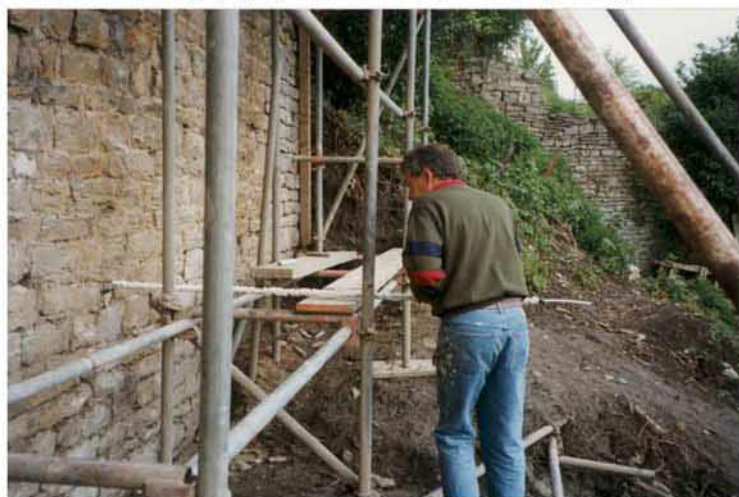
Diamond drilling (right) and anchor insertion (below).
