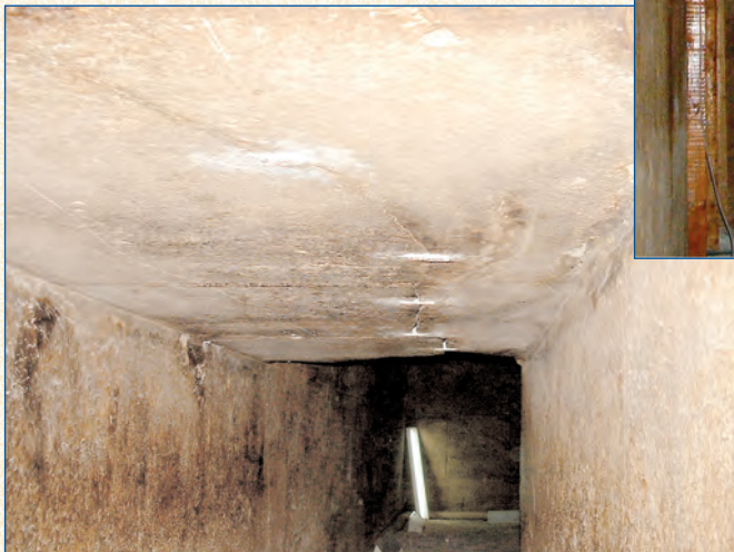
Soffit of cracked beam in the corridor between the burial chambers
