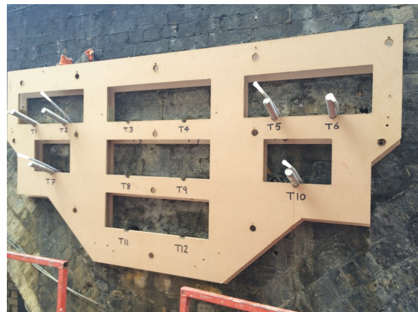
Above: A double template was adopted to ensure the precise alignment of the anchors in line and level and at the correct angle of inclination.
