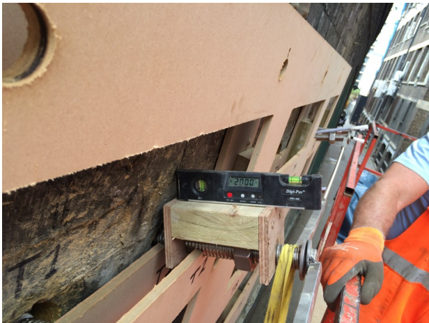
Above: Drilling was carried out by precise setting out of angles with a digital level at points determined by the engineers.
