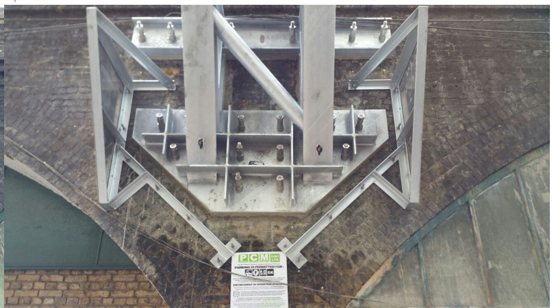
Above: The gantry base steelwork fitted perfectly without any need for adjustment due to the precision of setting out, alignment and installation of the anchors.
