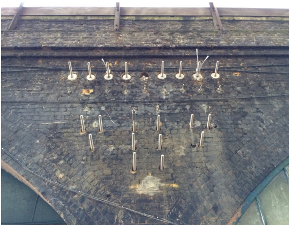
Above: the anchors installed awaiting the installation of the steelwork of the gantry base.
