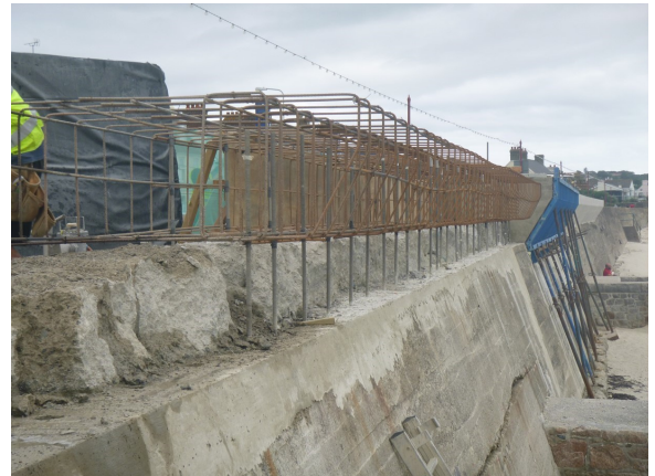
Right: new reinforcement added prior to concrete being poured.
