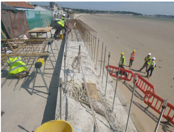
Left: Vertical anchors inserted prior to pouring.
