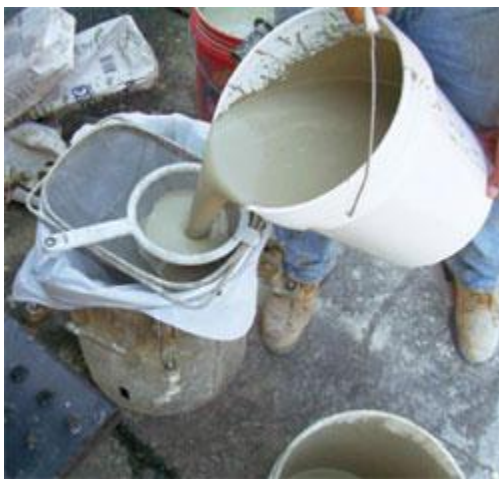
The masonry grout is strained to remove lumps before it is fed into the fabric sleeve.
