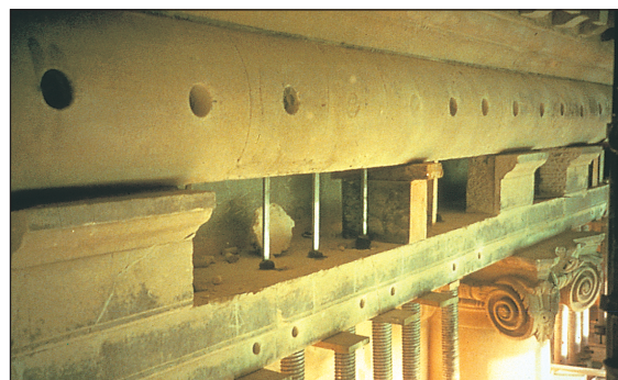
Entire length of 10 metres exposed
