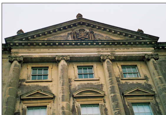
External upper beam area
