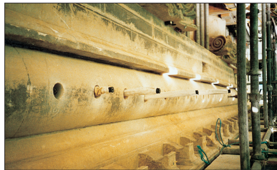
Anchor installation
