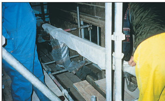
Insitu assembly of 100 x 100 mm stainless steel 10 m anchor
