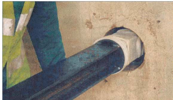
Insertion of Cintec section of 'I' beam into brickwork
