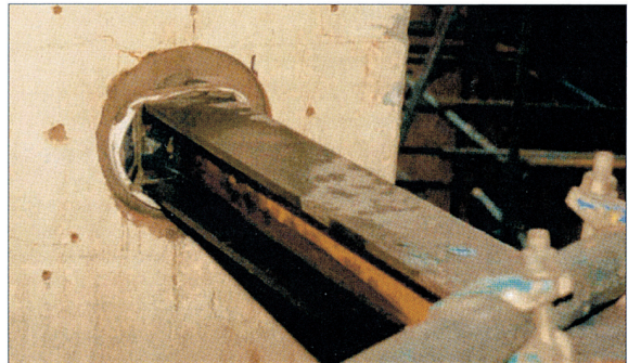
'I' beam following grout injection
