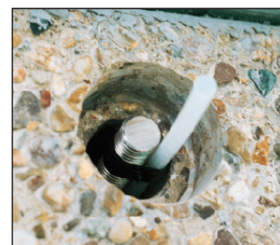
Anchor prior to injection
