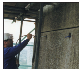
Injecting grout into anchor
