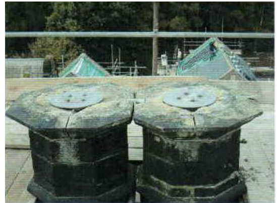
Chimney's capped with a stainless plate ->
