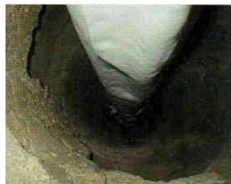
Partially missing ceramic liner ->
