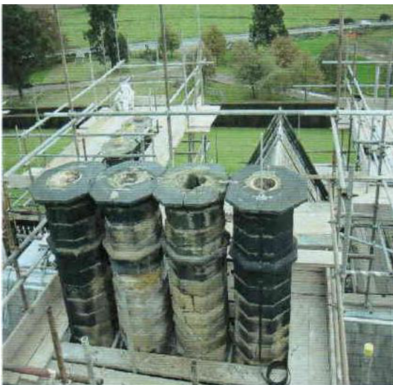
Partially missing ceramic liner ->
