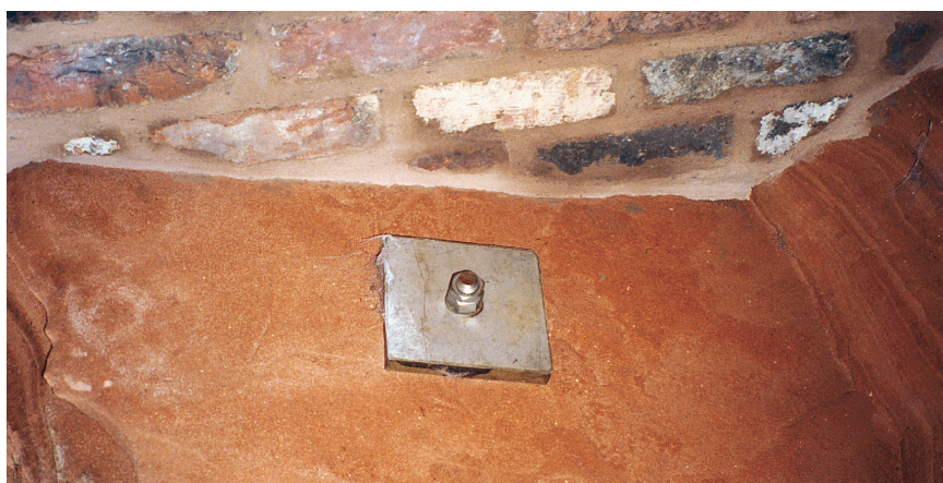
Roof bolt support to ballroom ceiling.
